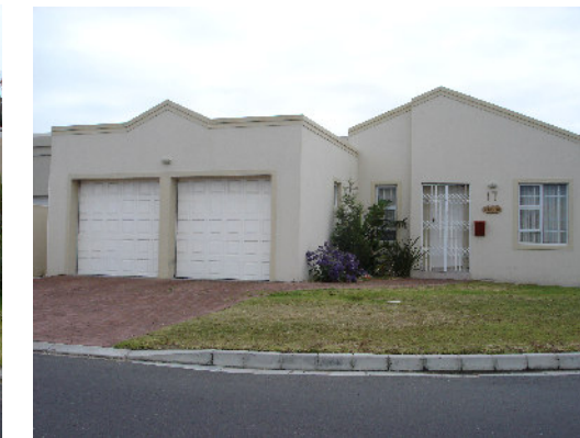
Cottage Style - double garage, but with central column breaking up the wide door facade.
