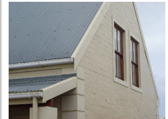
- Different architectural styles along a street length. - Note bagged wall finish with plaster bands
