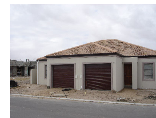
Terrace Style single storey
